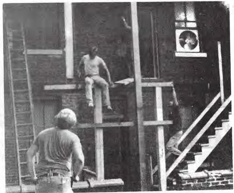
Mastermind Paul Lavella supervises porch construction
